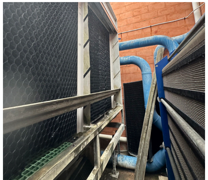
Work complete showing limited access and XF75IL Crossflow blocks installed
