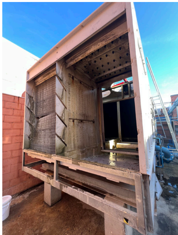
Work in progress shows old crossflow sheet fill being stripped from the cooling tower
