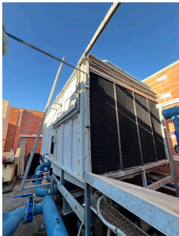
Cooling tower with old crossflow sheet fill prior to work commencing
