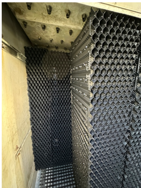
XF75 fill pack modular blocks during installation
